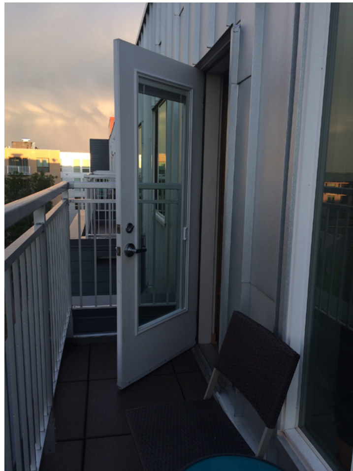
Figure 1—Example of balcony with no maneuvering clearance on the outside.
